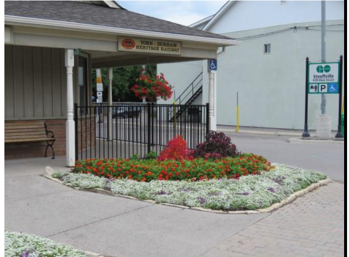
York Durham Heritage Railway Station
